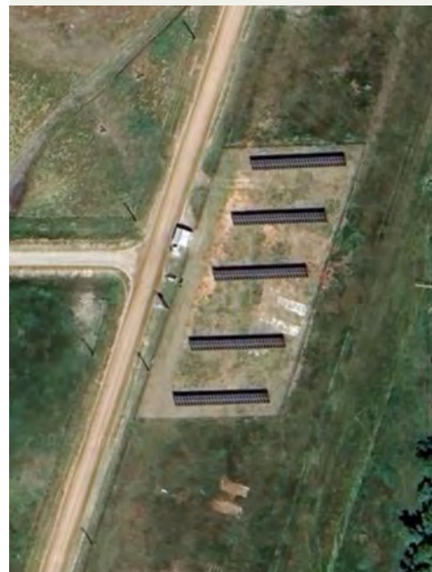
Hill Spring Irrigation Pump House Solar PV, Village of Hill Spring
